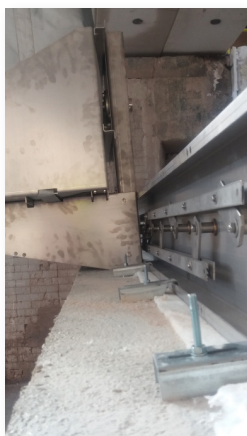
Close-up of fixed brackets and mineral fiber seal
